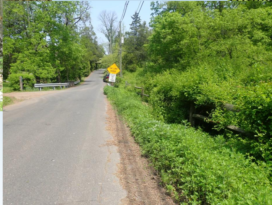
View of the east approach to the bridge
