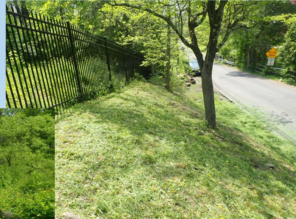
View from top of slope approaching the bridge
